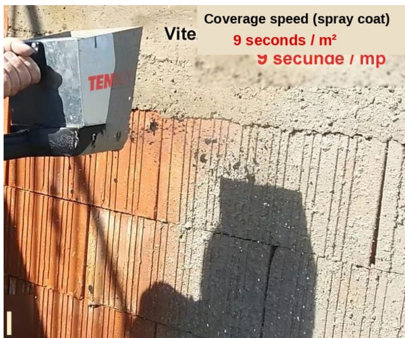
Figure 5. Example of applying the bonding / spray coat
