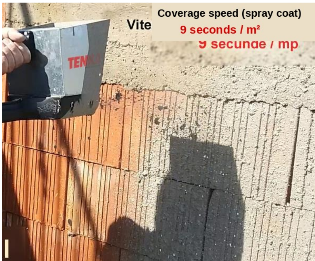
Pneumatic nozzle area during application
